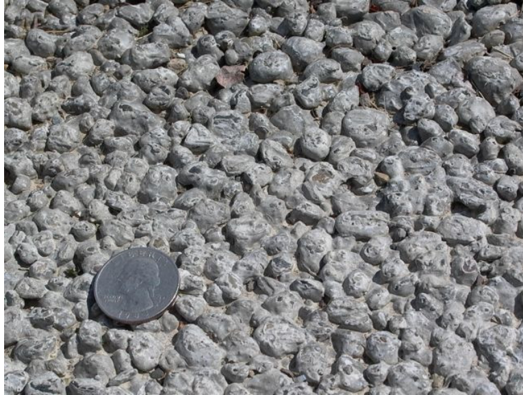
Figure PT-2.2: Porous concrete surface course in West Seattle, Washington. Quarter provided for scale. (Photo by J. Anderson)
