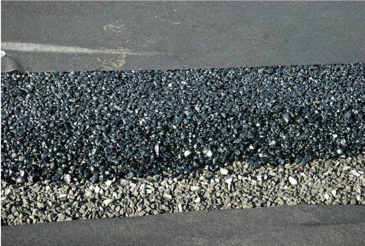
Figure PT-2.1: The appearance of porous asphalt is much the same as non-porous asphalt. The porous asphalt is placed over course of porous aggregate beneath a temporary geotextile fabric, which is to prevent clogging issues during construction. (Photo by K. Hansen, National Asphalt Pavement Alliance)
