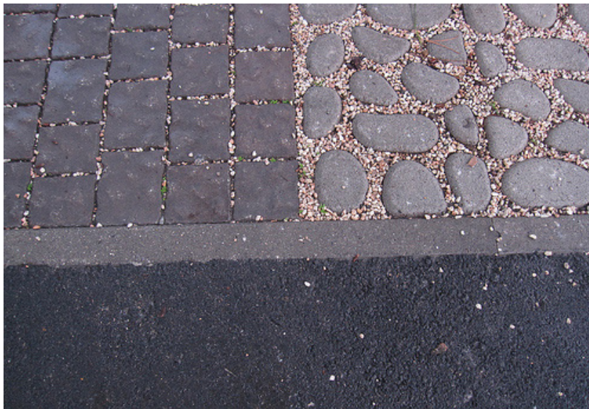
Figure PT-2.3: A variety of permeable pavers, bricks, and non-porous asphalt. (Photo by Sean Thayer)
